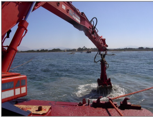
The bucked digger positioned on the pontoon used for the realization of the first part of the dig
