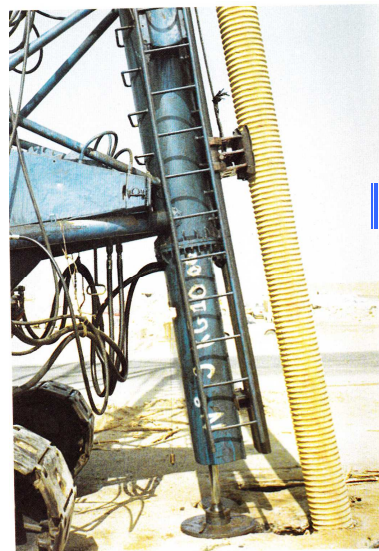
Insering the mandrel into the shell
