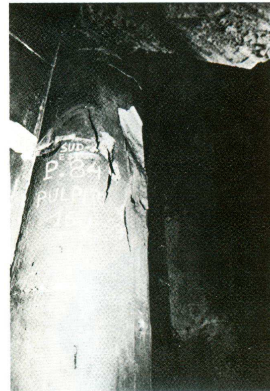
42.-43. The Milan Cathedral. Severe cracks in pylon 84 of the tiburium (1969).
